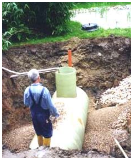
Figure 4.15. Urine tank and constructed wetland for treatment of greywater and leachate from the separation unit in Lambertsmühle.
