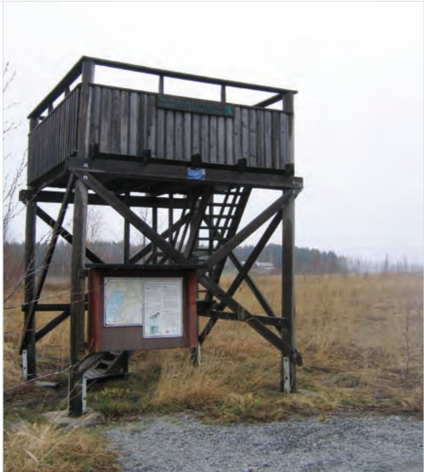
Bird observation tower built by the LIFE project
