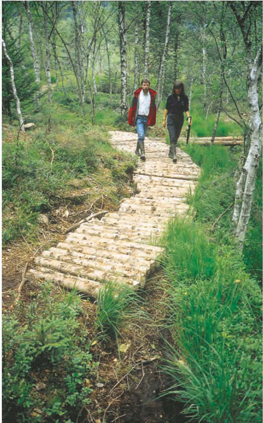
Boardwalk constructed through the Kendlmühlfilzen
