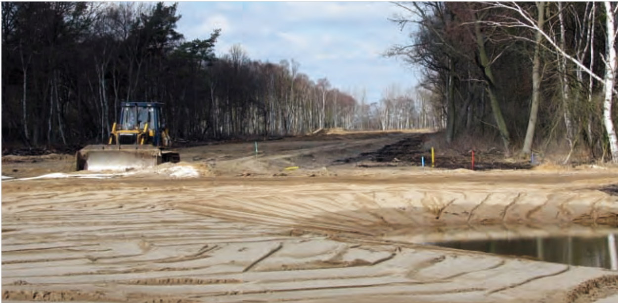
Clearing the surrounding area in order to build the dyke
