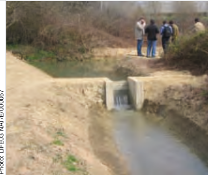
Restoration activities included the naturalisation of brooks and the restoration of ditches
