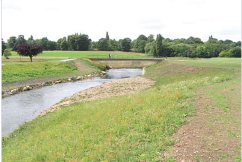
The banks of the river were lowered to allow the river to follow a more natural course
