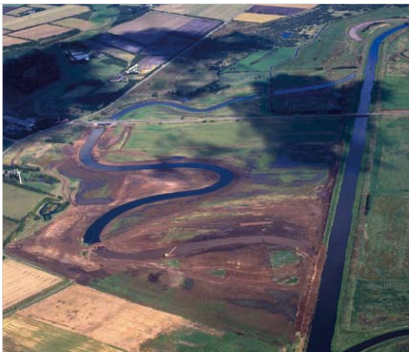
Aerial view showing the former straightened river section (right) and the re-meandered section during the construction period (left)
