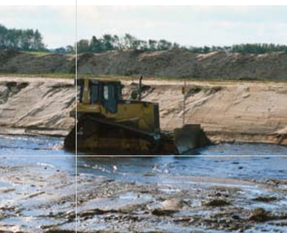
Reconstruction work on the River Skjern
