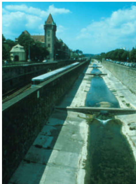
Figure 2 Downstream section of the Wienfluss at low water level and during the flood event of 1992. Due to the geological situation in the catchment area (Viennese sandstone, Flysch) there are great differences between low and high water levels.
