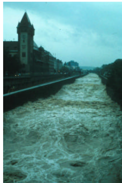
Figure 2 Downstream section of the Wienfluss at low water level and during the flood event of 1992. Due to the geological situation in the catchment area (Viennese sandstone, Flysch) there are great differences between low and high water levels.
