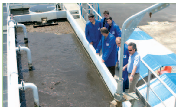
Practical work on a pilot unit for wastewater treatment with activated sludge
